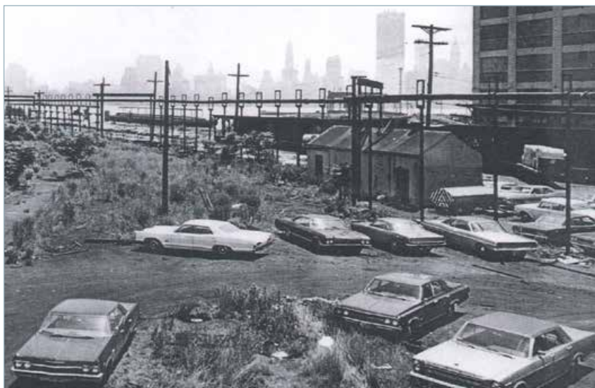
The decline of rail commerce on the Jersey City waterfront left the neighborhood that would later become known as Newport underutilized. The infusion of $75 million in grants and financial assistance for site preparation and infrastructure replacement subsequently catalyzed redevelopment in Newport.
